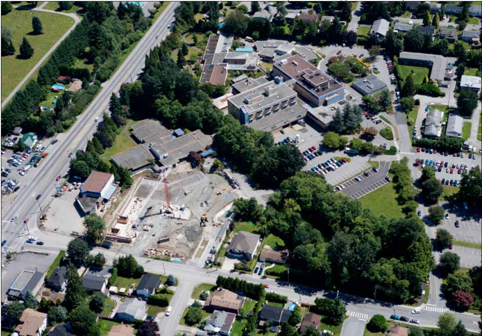
Baillie House, a new hospital building, coming out of the ground on the north side of McKenney Creek. If the footprint had of been moved 40 to 50-feet to the south, there was a chance that the new McKenney Creek Hospice Residence could have had access to lawns and the creek.
