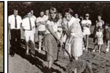
July 1985: Official sod turning prior to school construction.
