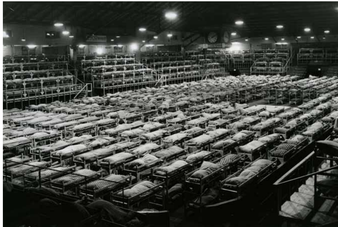
HASTINGS PARK CLEARING STATION 1942. Building K, formerly the Forum, was turned into the Japanese men's dormitory. The Park was taken over by the BC Security Commission to temporarily house and disperse the Japanese Canadians in the early months of 1942. This photo was taken by Leonard Frank, a well-known Vancouver commercial photographer who was hired by the BC Security Commission to document the clearing station and the camps.
